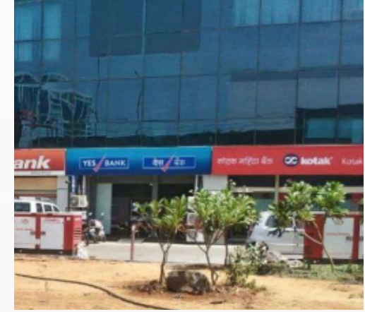
Leading Partner for the Banking Sector 5 kVA to 500 kVA x 4000
